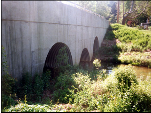
Figure 13 Multiple-cell culvert constructed with two cell inverts at bankfull elevation.
