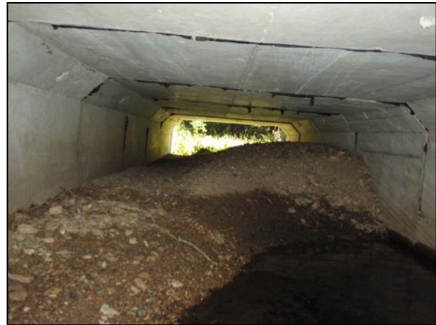
Figure 10 Extensive deposition of sediment within one of the cells of the culvert.
