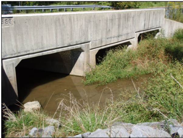
Figure 9 Typical view of the three-cell box culvert across an unnamed tributary to Little Bennett Creek, Maryland.
