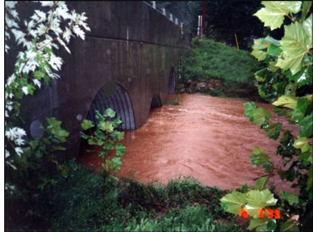
Figure 14 The multiple-cell culvert in Figure 13 performing at high flow.
